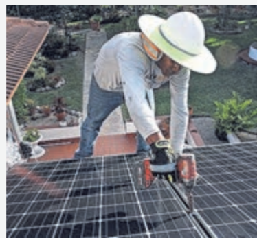
Climate change is shaking up insurance coverage, and blazes in California this year have led underwriters to tighten terms for solar projects — Jose Carlos Fajardo/Bay Area News Group/San Jose Mercury News via AP
